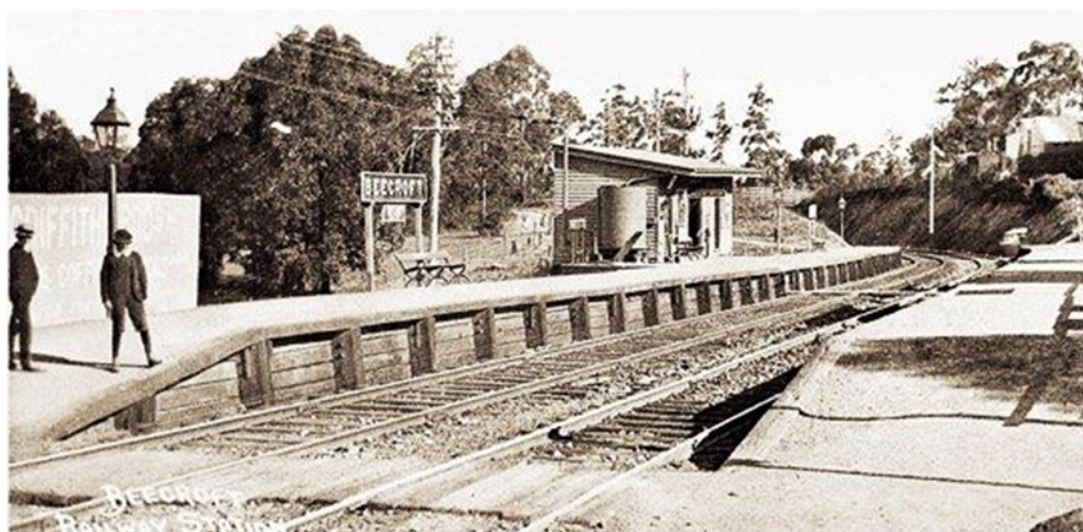
Beecroft Station around 1910 looking south, here with two lines and separate platforms. There is a rainwater tank on the waiting room, lamp (kerosene?), signals and top right the stationmasters house. At this stage there was a ladies toilet on the down station. Note the boards of the walkway between the platforms. [Hornsby Shire Recollects]
