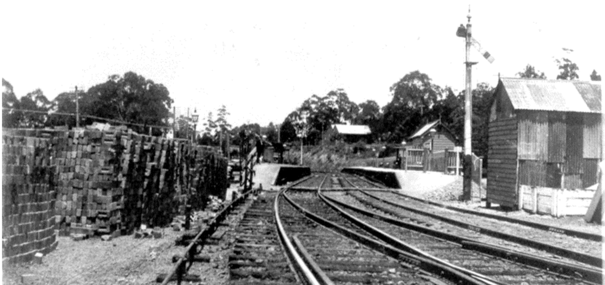
Beecroft rail station around 1912? with two platforms, prior to rebuild as an island platform. Bricks for construction at left. Distance centre shows the old stationmasters house in what is now a reserve and behind the Cenotaph. Points for the goods siding can be seen. [HSR; Norma Macdonald].
